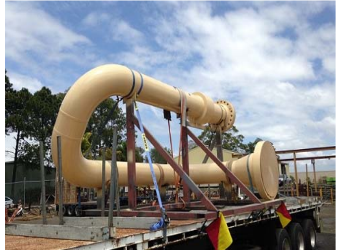
High Pressure Gas Tie In Pipe Spool - GLNG
