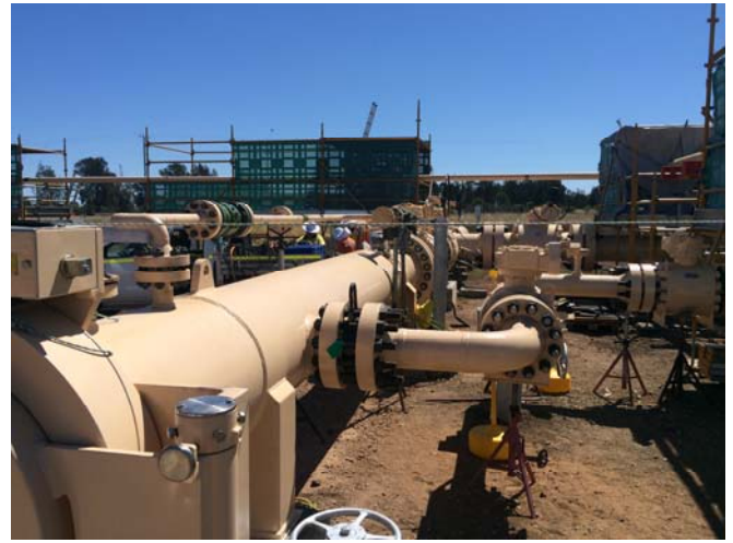
High Pressure Gas Piping Installation - GLNG
