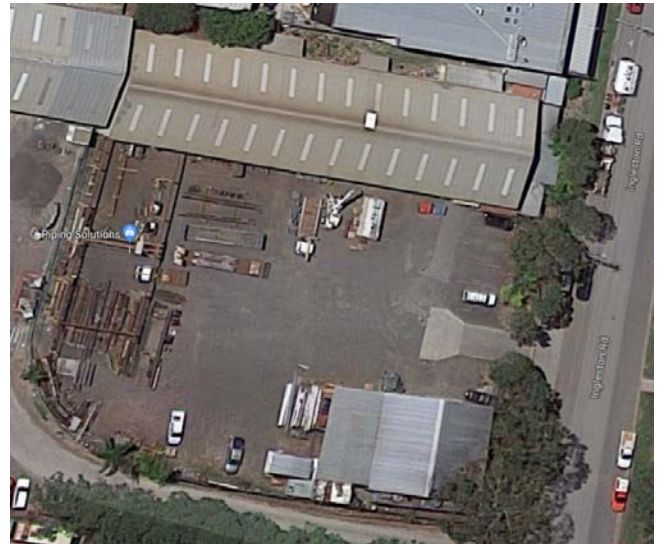
Piping Solutions Workshop 1 1/107 Ingleston Rd, Wakerley
