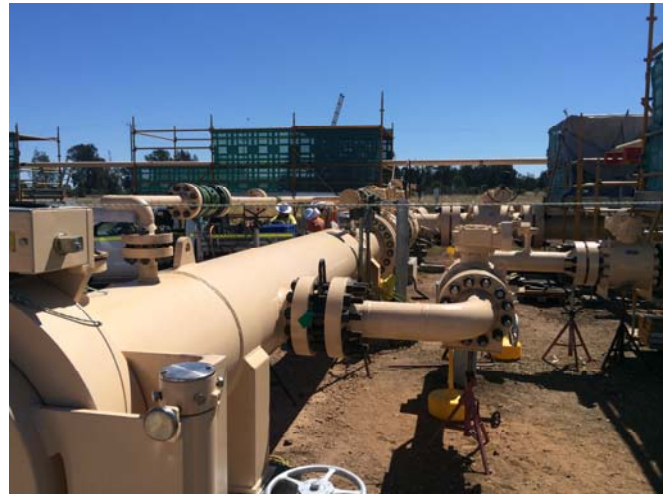
High Pressure Gas Piping Installation - GLNG
