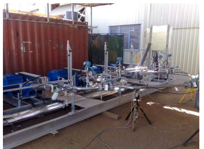
Co2 Compressors Skid - Gas Technology
