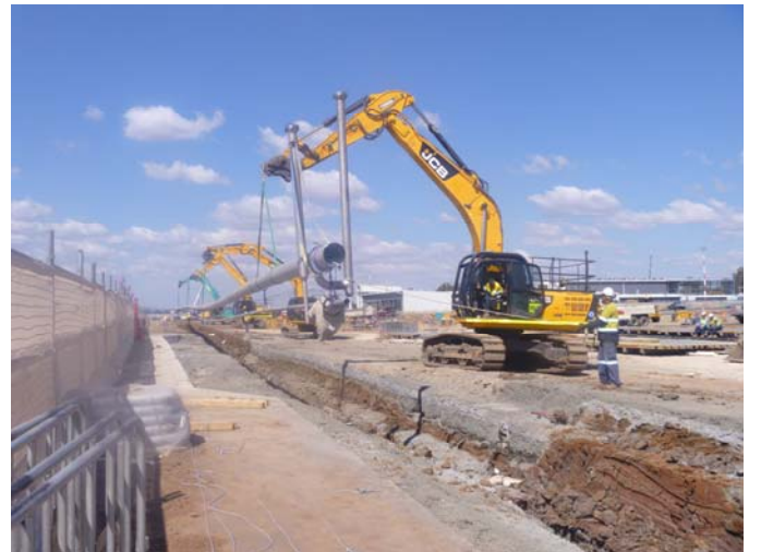
4 Crane Lift – RAAF Amberley
