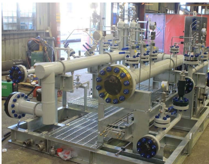
Oil / Gas Wellhead Metering Skid - Oil Search
