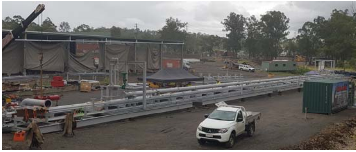
Skid Pipe Work Compressor Station – Wasco / Senex
