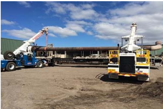
Dual Lift of 600nb Sch160 x 24m Pipe Spool - GLNG
